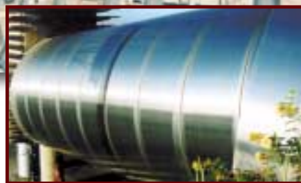
Aeroporto Fortaleza, Fortaleza, Brazil Architect: Claudio Silva, 1997 Stainless steel panels bonded to steel frame.
