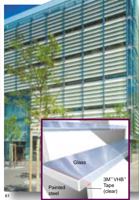
Glass steps bonded to varnished steel frame, Tamedia Building, Zurich, Switzerland
